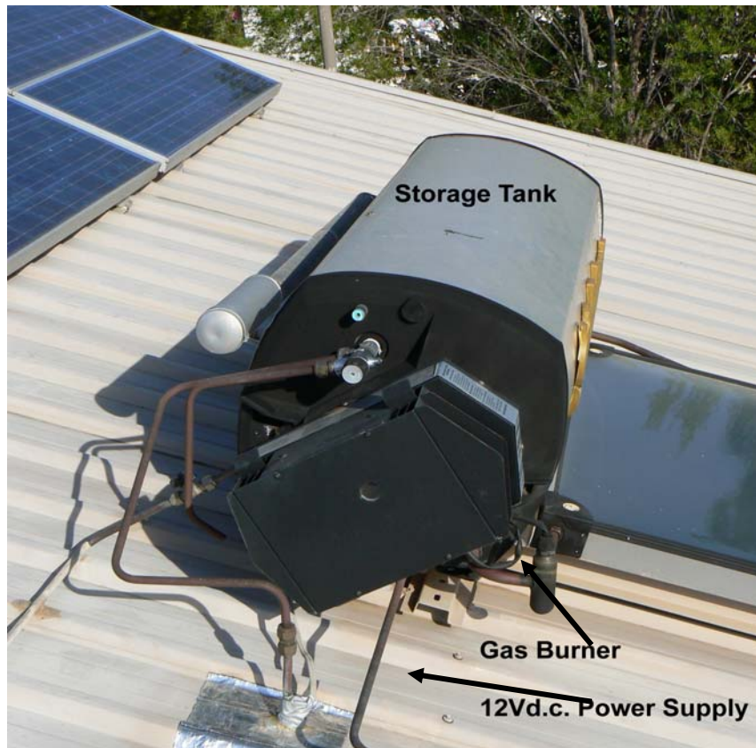
Figure 4.1.5 – Tank-mounted gas booster
