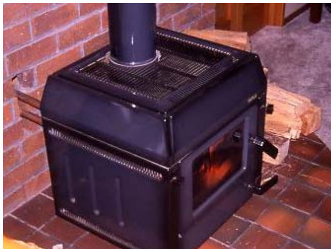
Figure 4.2.3 – Wood heater with boiler coil
