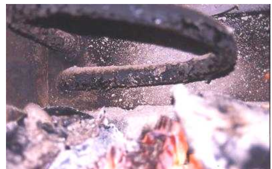
Figure 4.2.3 – Wood heater with boiler coil
