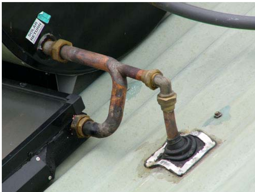
Figure 4.2.12 – Roof penetration for heat exchanger
