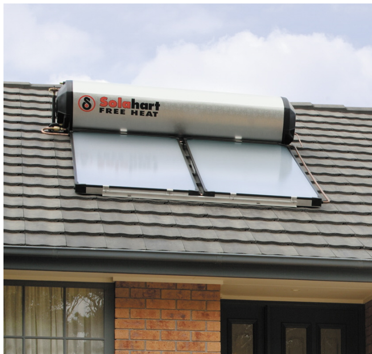
Figure 3.4.1 – Typical close coupled system and components
