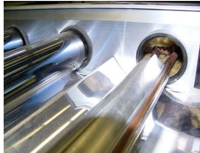
Figure 3.2.6 – Constructions details for a U-tube type evacuated tube collector
