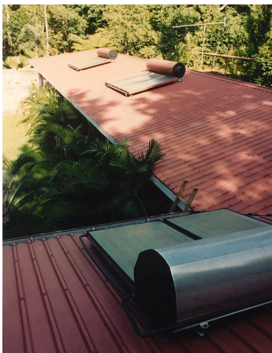
Figure 2.2.2 – Extreme shading of solar hot water systems
