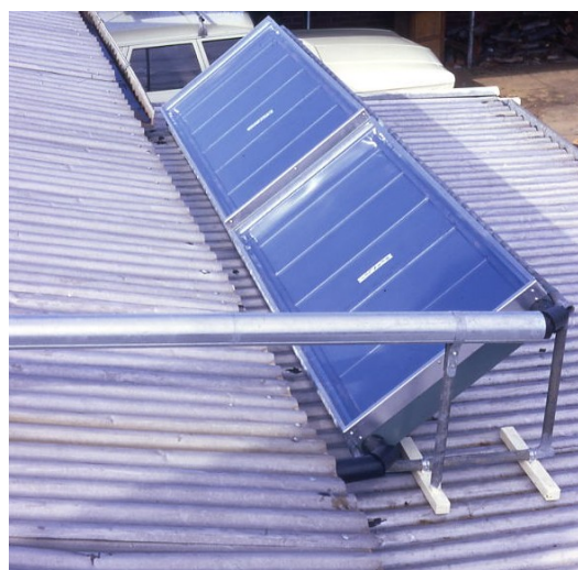
Figure 2.2.1 – Partial shading of collectors from chimneys and interconnecting pipes
